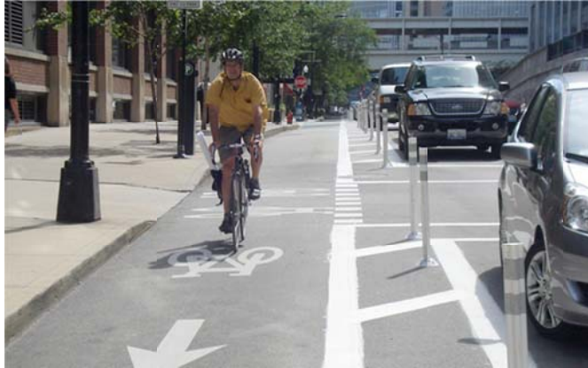
Option 5: Protected Bike Lane/Cycle Track (with a physical barrier between the bike lane and motor vehicle travel lane)
