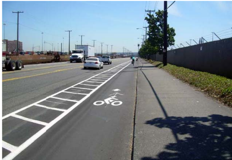
Option 4: Buffered Bike Lane (painted buffer between bike lane and motor vehicle travel lane):
